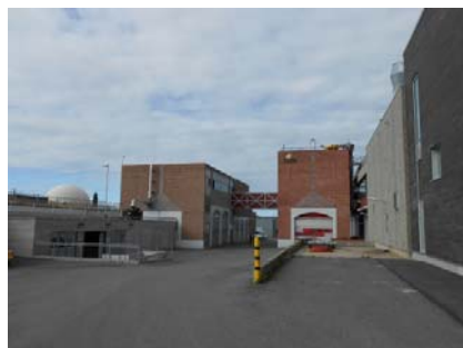
HIAS Sewage Treatment Plant
